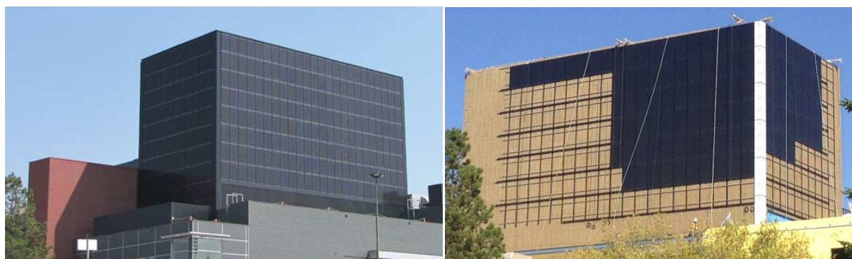
Figure 15: a and b: Arts Centre building (a); Integration of PV modules as BIPV cladding (b). (Photo credit: Gordon Howell).
