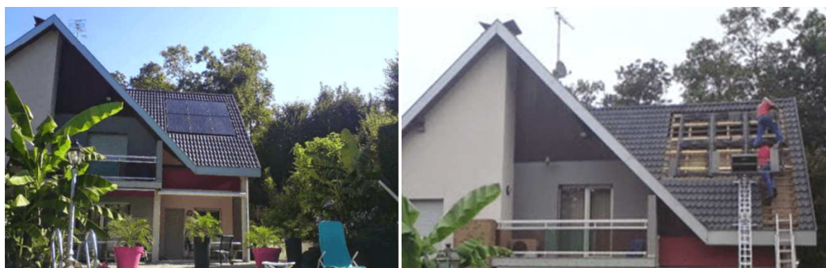
Figure 9: a and b: Altkirch house (a); Integration of the BIPV-T panels (b) (Dualsun, 2019).
