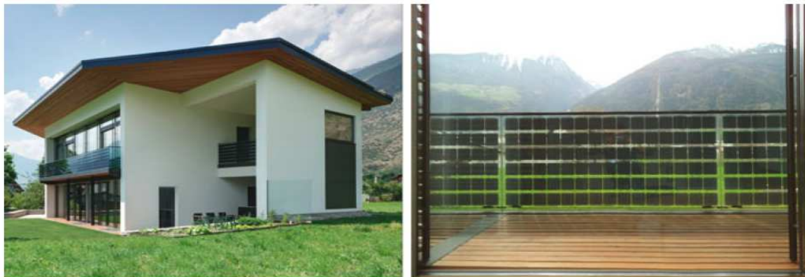
Figure 23: Lasa house (a); BIPV balustrade layout (b) (Photo from Maturi and Adami 2018).
