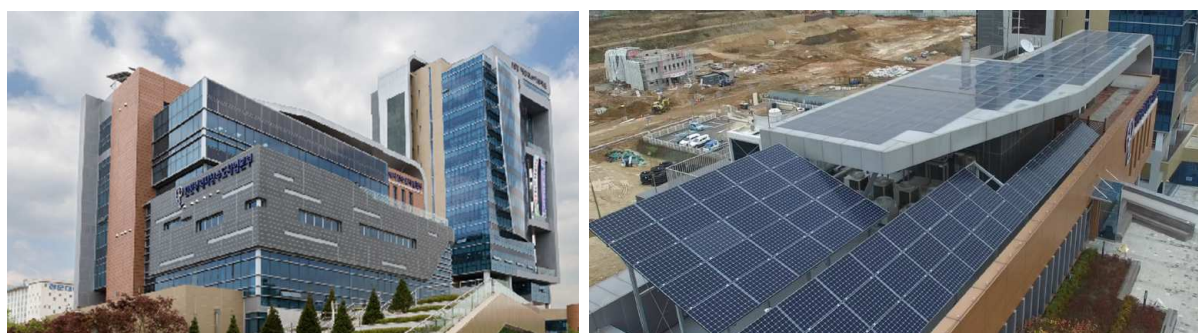
Figure 5 a and b: Public Town building (a); BIPV roof (b).
