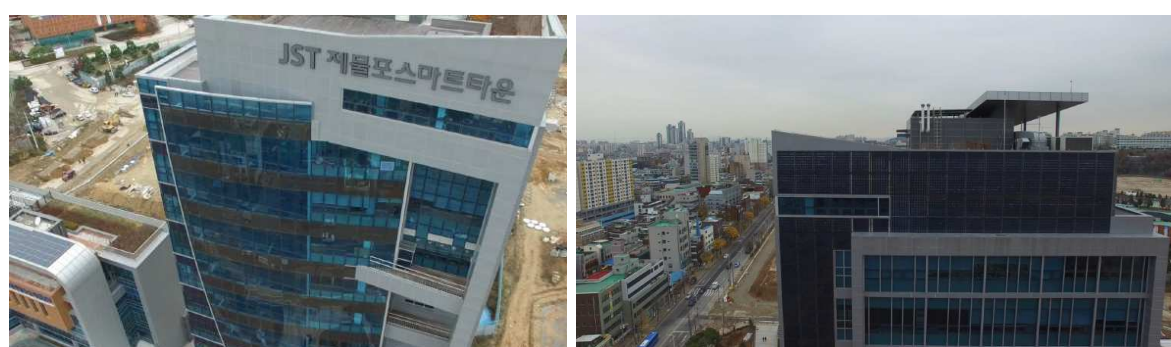
Figure 13: a and b: JST building (a); East façade BIPV (b).
