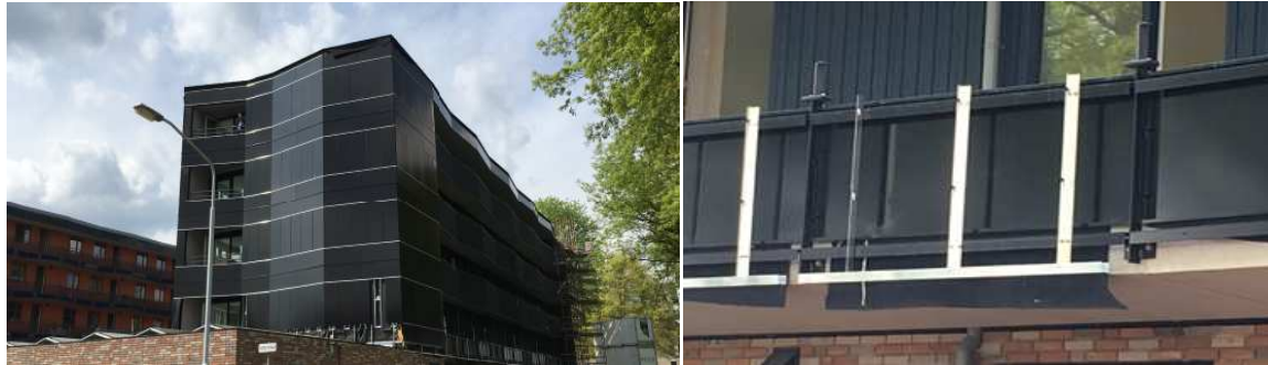
Figure 17: a and b: De Willem de Zwijger buildings (a); BIPV mounting system (b).
